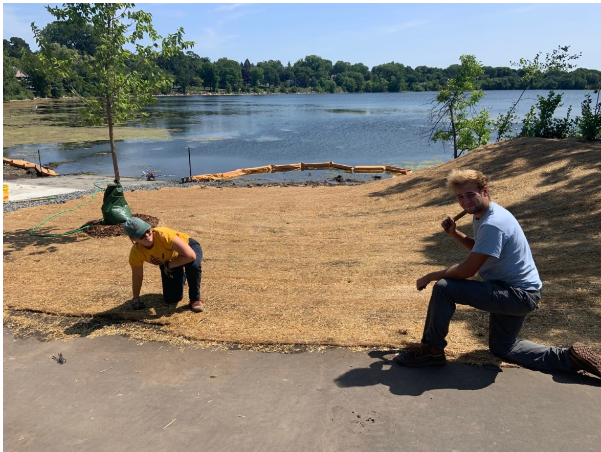
At the new Lake Phalen boat ramp, interns Mike and Emily stapled down biodegradable erosion control blanket after we broadcast a short grass prairie seed mix and an oats cover crop. Aggressive shoreland plant species like prairie cord grass, lake sedge, and Canada blue-joint were installed at the Normal Water Level.
