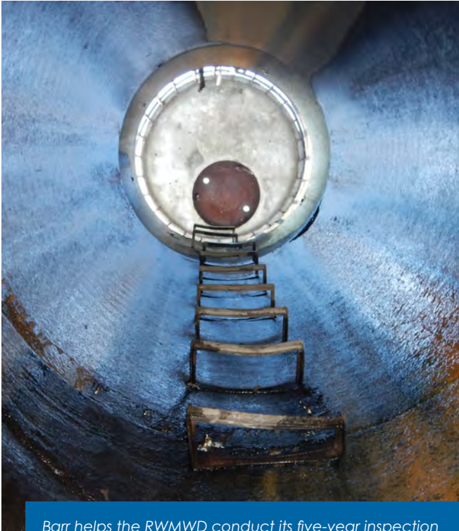
Barr helps the RWMWD conduct its five-year inspection cycles for the Beltline and Battle Creek storm sewers to keep up to date on the maintenance needs of these important conveyance systems. This photo was taken from the bottom of the Battle Creek storm sewer, looking up at one of the creek's several overflow structures that Barr designed in the 1980s.
