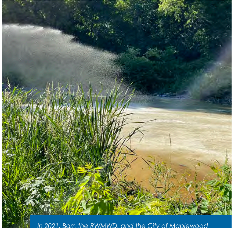
In 2021, Barr, the RWMWD, and the City of Maplewood partnered on a research project funded through the University of Minnesota's Stormwater Research Council that involved applying spent lime in a slurry form to a pond south of Wakefield Lake. The goal of the project was to determine whether spent lime can decrease the internal load of phosphorus from the pond's sediments.
