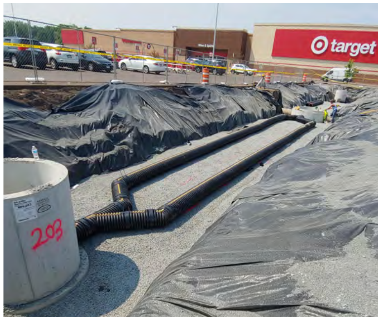
Over the past few years, Barr assisted the RWMWD in the design and implementation of stormwater retrofit and green infrastructure features at two City of Saint Paul Target stores. The projects included removal of impervious parking spaces, installation of infiltration rain gardens, and construction of tree trenches. This photo shows the underdrains for one of the tree trenches constructed in the parking lot of the North Saint Paul Target site.
