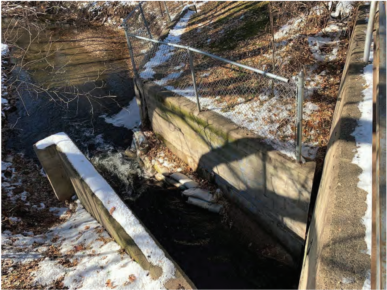
Downstream exit of culvert
