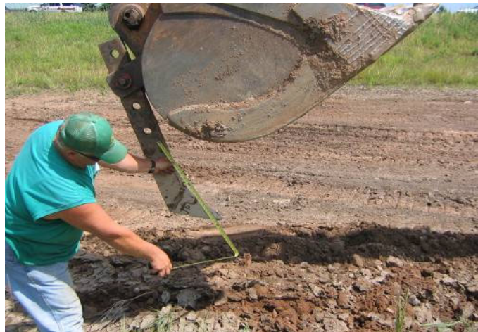
Photo caption: A variety of equipment is available to rip soils including backhoe with ripper, backhoe without ripper, and hydraulic spade.
