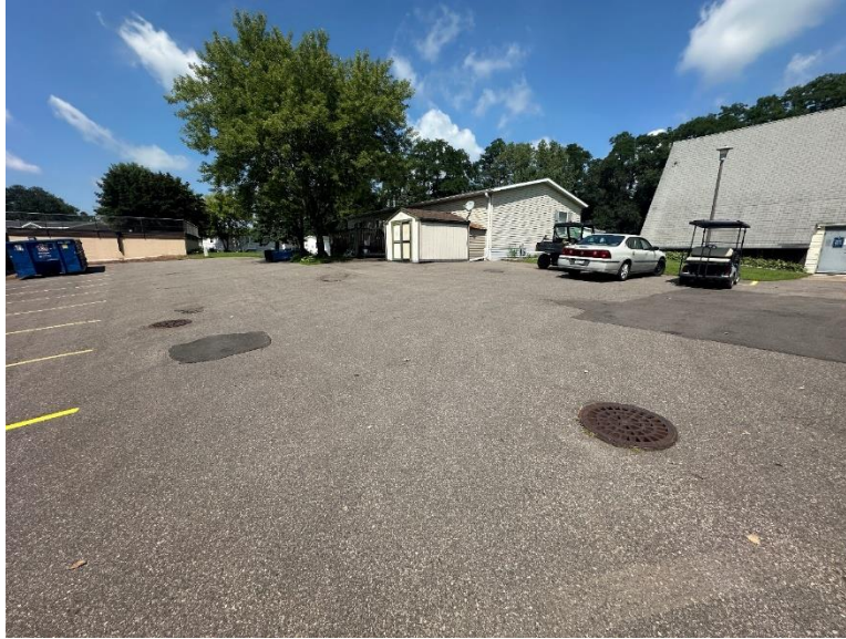
Photo 8: Parking lot with storm manholes that surcharge during large rain events
