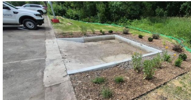
Completed pretreatment structure at Maplewood Toyota. At top, pre-curb modification. At bottom, post-curb modification (see change order for more information).
