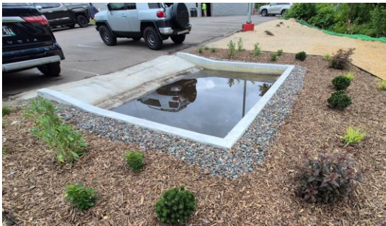
Completed pretreatment structure at Maplewood Toyota. At top, pre-curb modification. At bottom, post-curb modification (see change order for more information).
