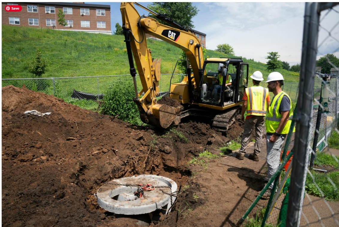
A construction crew adds a manhole to connect floodwater drainage to a main sewer line near Roosevelt Homes in St. Paul. (Renée Jones Schneider/The Minnesota Star Tribune)
