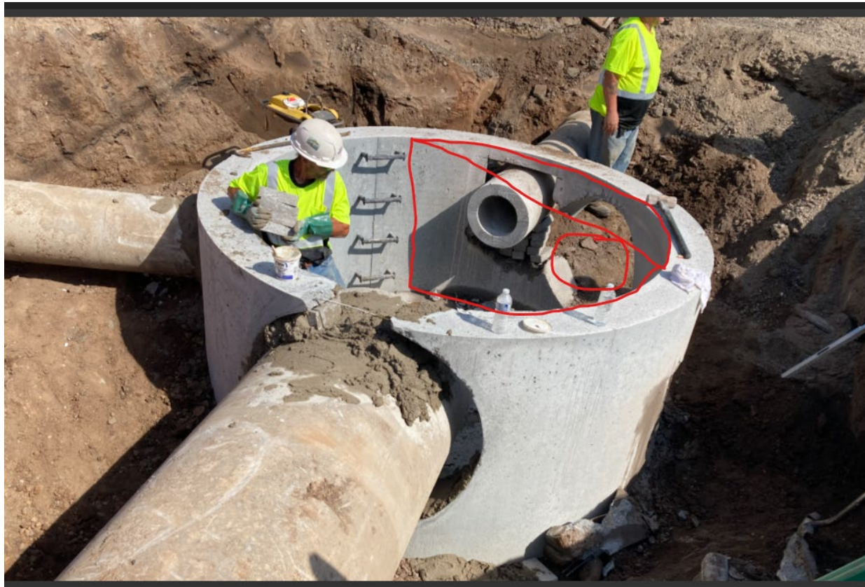
Figure 3 – Image from 7/15/2025 showing MH-2 configuration in the field. Note the red markup where concrete shall be installed in addition to the City Standard Plate sewer bricking and mortar.
