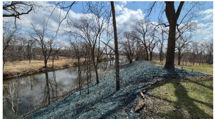
Keller Creek Slope (T-B) 1. Before 2. Mopping up after burn 3. After installation of seed mix with hydromulch
