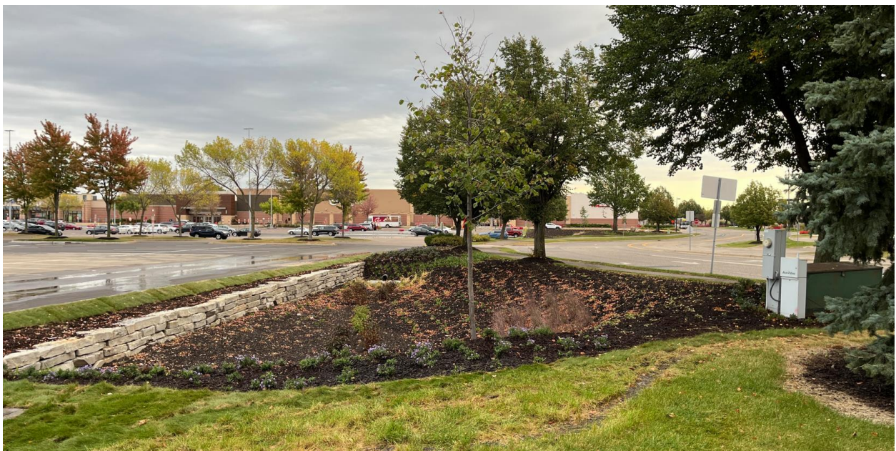
Figure 1: The completed south filtration rain garden at the Woodbury Target
