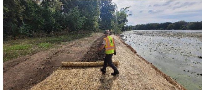
Keller Shore Phase 2 Install- top to bottom: Installing biologs, jetting in rock, rolling out erosion control fabric.
