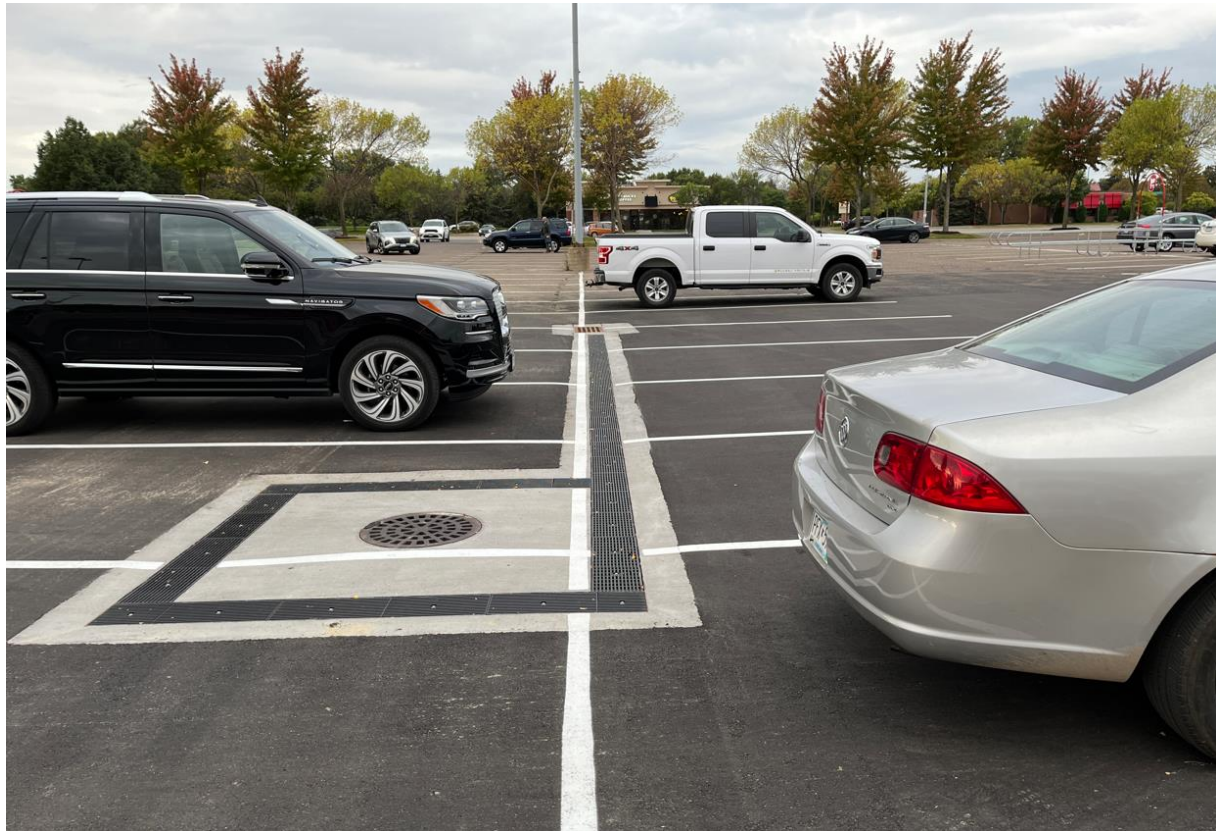
Figure 2: The completed trench drains that will collect runoff in the north parking lot and direct to the north filtration rain garden for treatment
