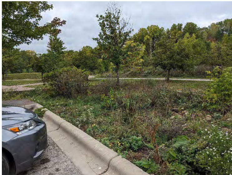
Image 5 - Infiltration basins at Eastside Heritage Park collect stormwater runoff from adjacent parking lot.
