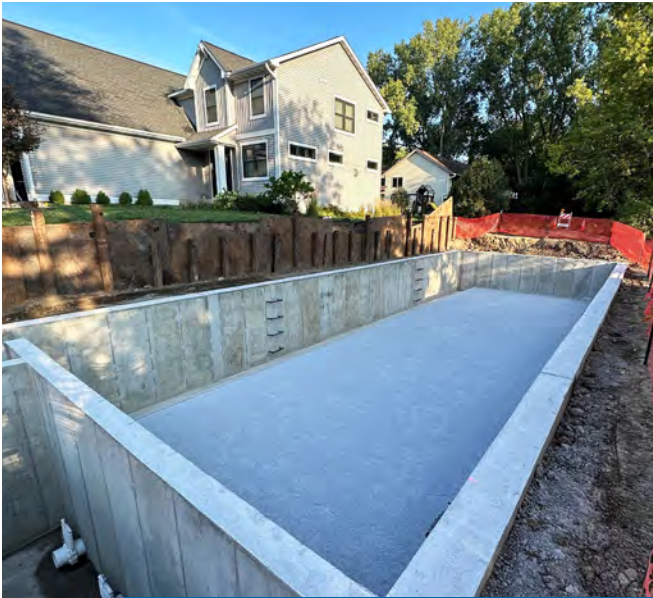
This regional stormwater BMP in the Lake Emily subwatershed helps decrease phosphorus loads to Lake Emily, which is at risk of impairment from excess nutrients. The unique underground filter system utilizes crushed limestone to inactivate the phosphorus and improve the lake's water quality. Barr helped the district assess alternatives and design the treatment system, and we coordinated construction on the RWMWD's behalf.
