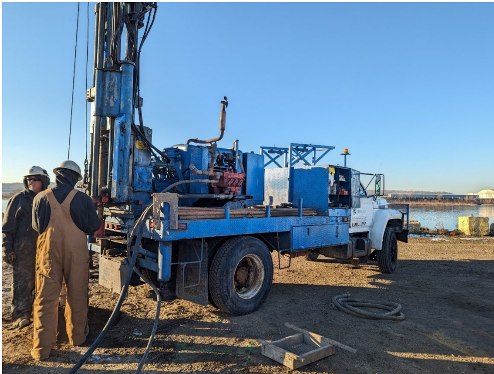
Figure 2-1 Geotechnical boring
