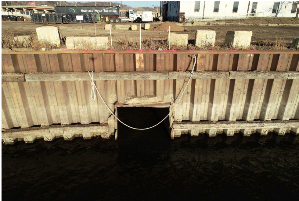
Figure 2-2 Drone survey of the existing outfall
