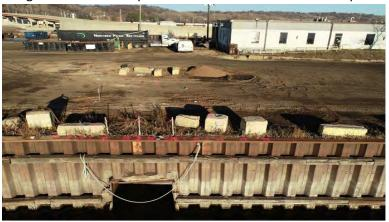
Drone photo of where the Beltline tunnel meets the Mississippi River through a river wall owned by St. Paul Port Authority. The concrete blocks in the background show the manhole location, which is the upstream limit of the proposed tunnel replacement.
