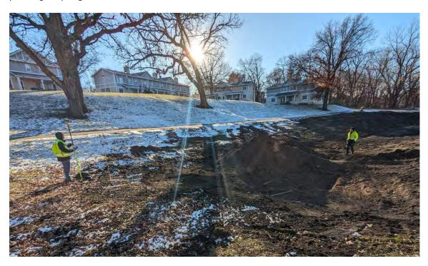
Construction of stormwater improvements began at Roosevelt Homes at the end of November. The photograph shows Barr and District staff checking final grades at the expanded stormwater basin. The additional storage volume will reduce flood risk for the area adjacent to the basin and allow for additional stormwater system modifications on the property to remove habitable structures from the floodplain.
