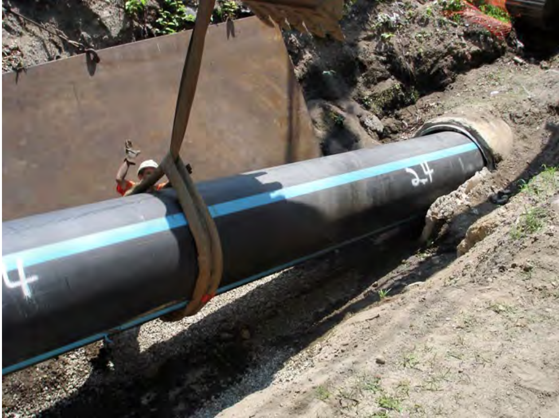
Figure 3-1 Slip Lining
