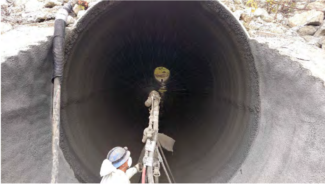
Figure 3-4 Spincast/Shortcrete Liner
