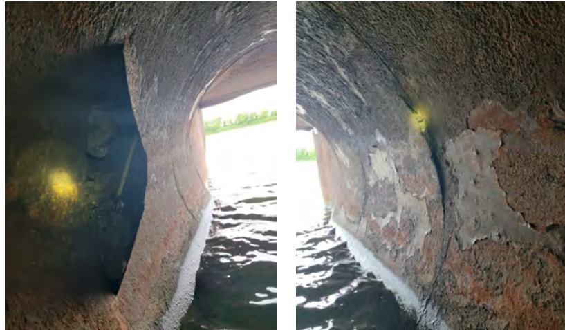
Figure 1-2 Deformation and Joint Separations in 9-foot Diameter Steel Pipe
