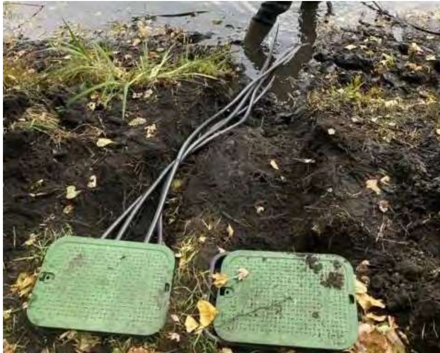
Two splitter boxes were installed on the pond shore. Four hose lines exit each box and run air to the diffusers.
