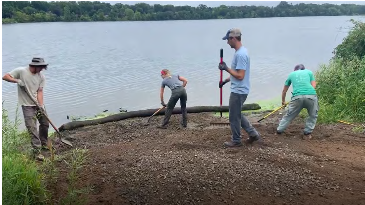
NR staff restored the old Lake Phalen boat ramp (concrete slabs were removed last year). The soil was mechanically tilled, a gravel layer was redistributed, and then covered with a compost-soil mixture.
