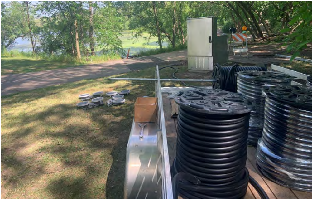
1,800' of weighted hose is being used to send air to the diffusers.
