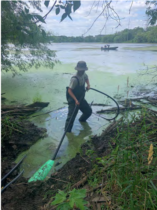
Hose being pulled under the path and then positioned offshore by a crew in a johnboat.
