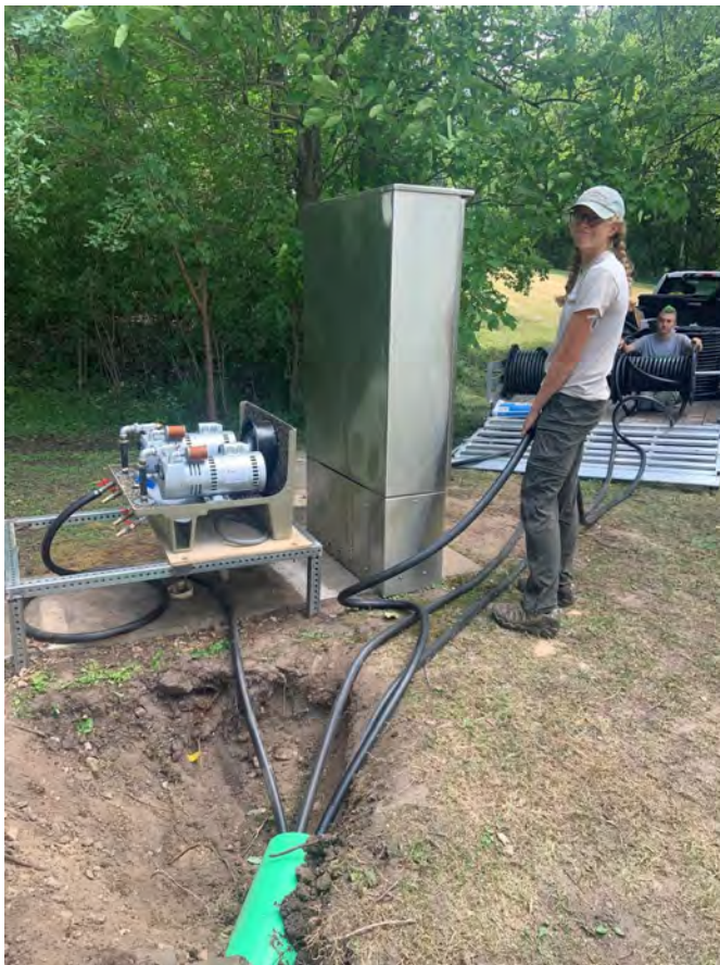
¾" hose being fed under the walking pathway, and then fastened to the pump stems.
