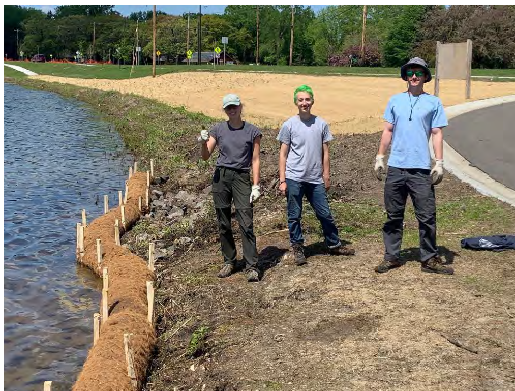
Our NR intern crew installed erosion control materials – coconut biologs and blanket.
