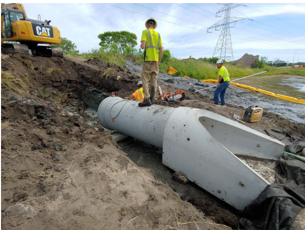
August 19, 2020, facing southeast: The contractor is shown installing the flared end section in the MnDOT stormwater pond, which has been dewatered to allow for outlet installation. Following construction, the flared end section will be below the normal water level of the pond.
