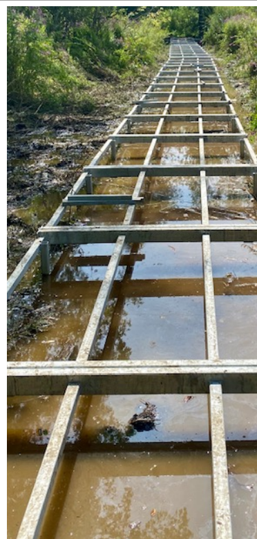
Boardwalk in progress
