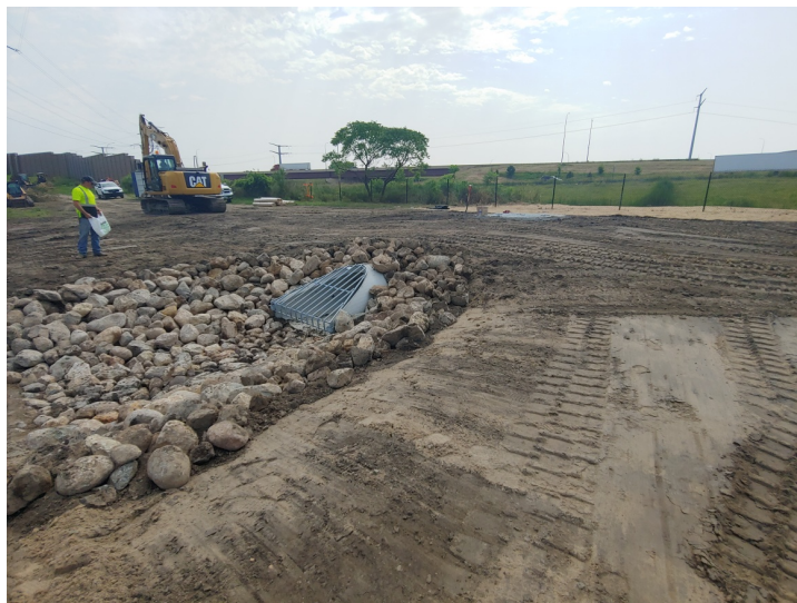
August 19, 2020, facing southeast: The contractor is shown installing the flared end section in the MnDOT stormwater pond, which has been dewatered to allow for outlet installation. Following construction, the flared end section will be below the normal water level of the pond.
