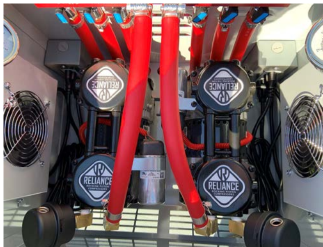
Two compressors feed air to the diffusers on the pond bottom.
