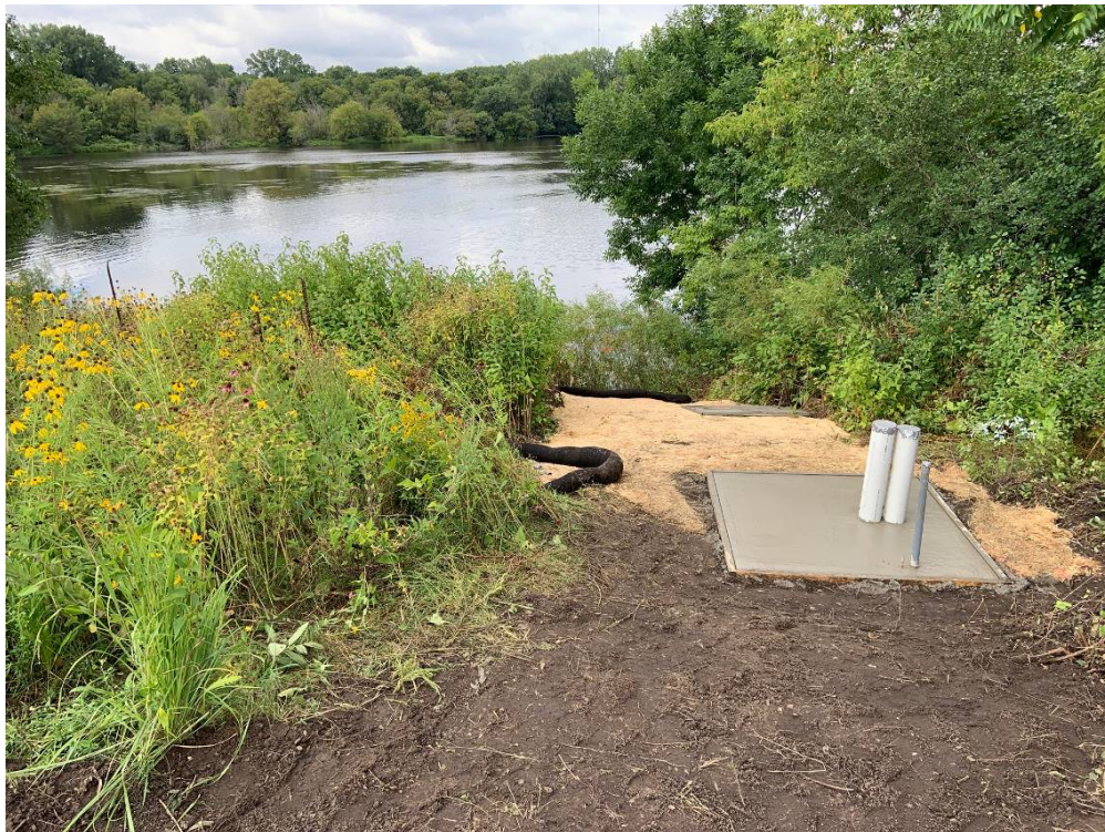
A concrete pad with power was installed to support the aeration unit. Hoses will be run in the PVC pipes down to the water's edge and then out to the center of the pond.
