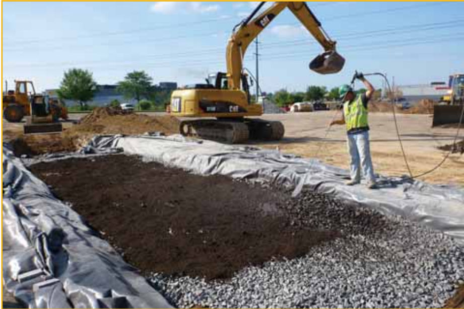
Above: Tree trench with side wall filter fabric (also gets wrapped over the top of the trench), first course of rock, and perforated pipe. Below: Top layer of rock with soil being washed into rock.
