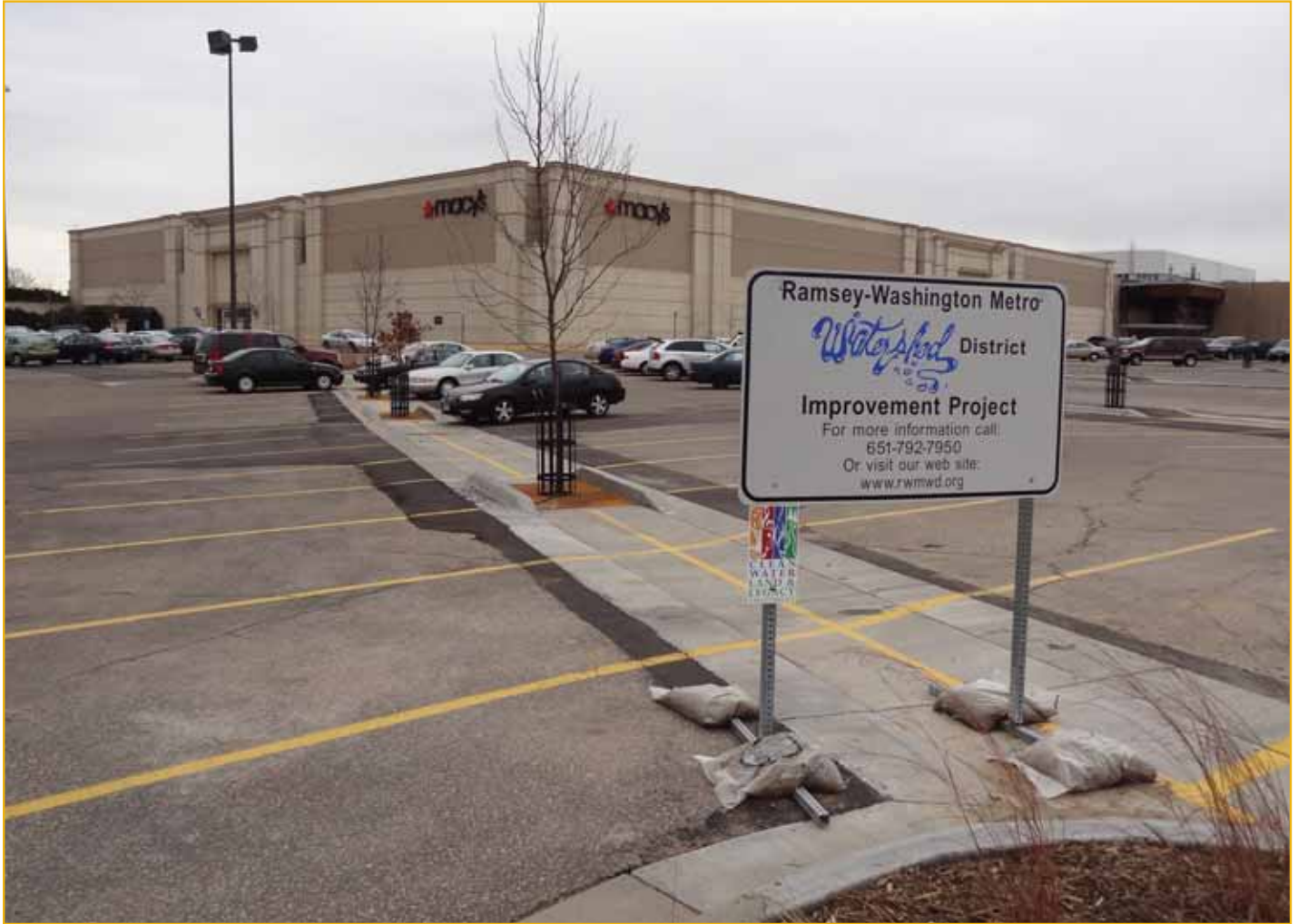
Completed tree trench in Northwest tree grove (Spring 2012).
