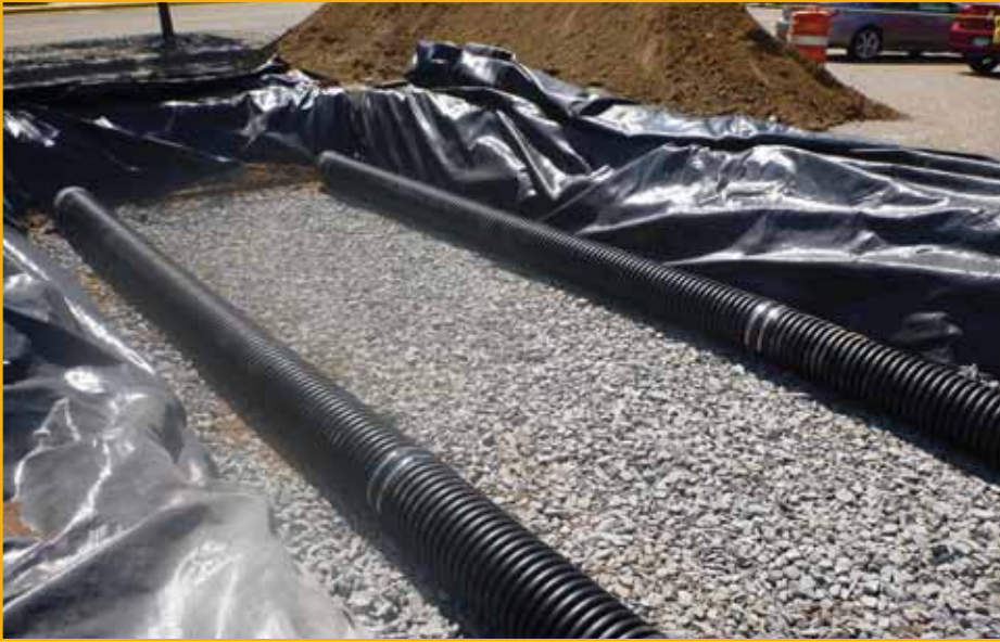
Above: Tree trench with side wall filter fabric (also gets wrapped over the top of the trench), first course of rock, and perforated pipe. Below: Top layer of rock with soil being washed into rock.
