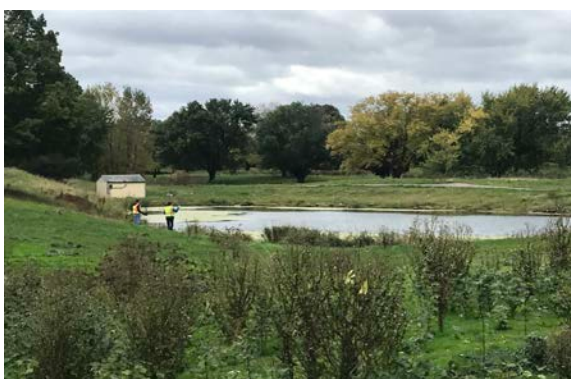
Team members inspect a pond that collects local
