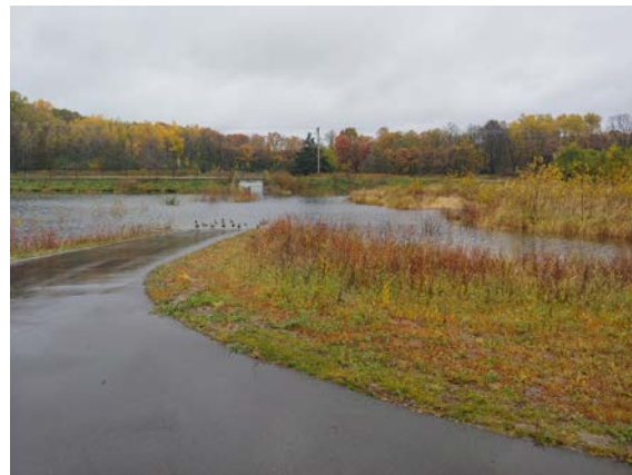
Looking north toward the stop logs at the pedestrian tunnel on October 22, 2019
