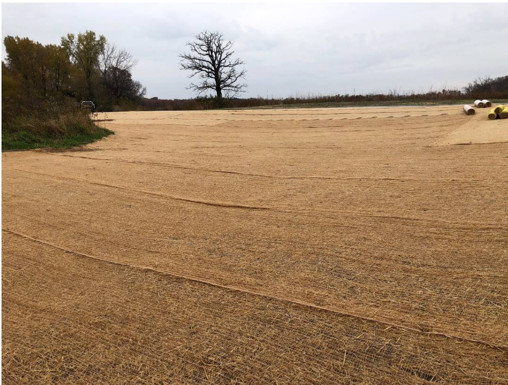
After re-grading, re-seeding and blanket installation
