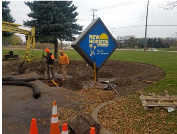
Construction of the rain garden at the New Horizon day care in Woodbury
