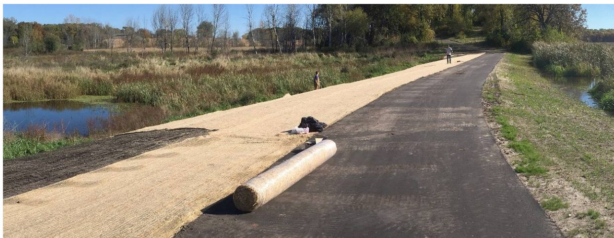
A heavy duty straw-coconut fiber blanket will protect the slope over the winter.
