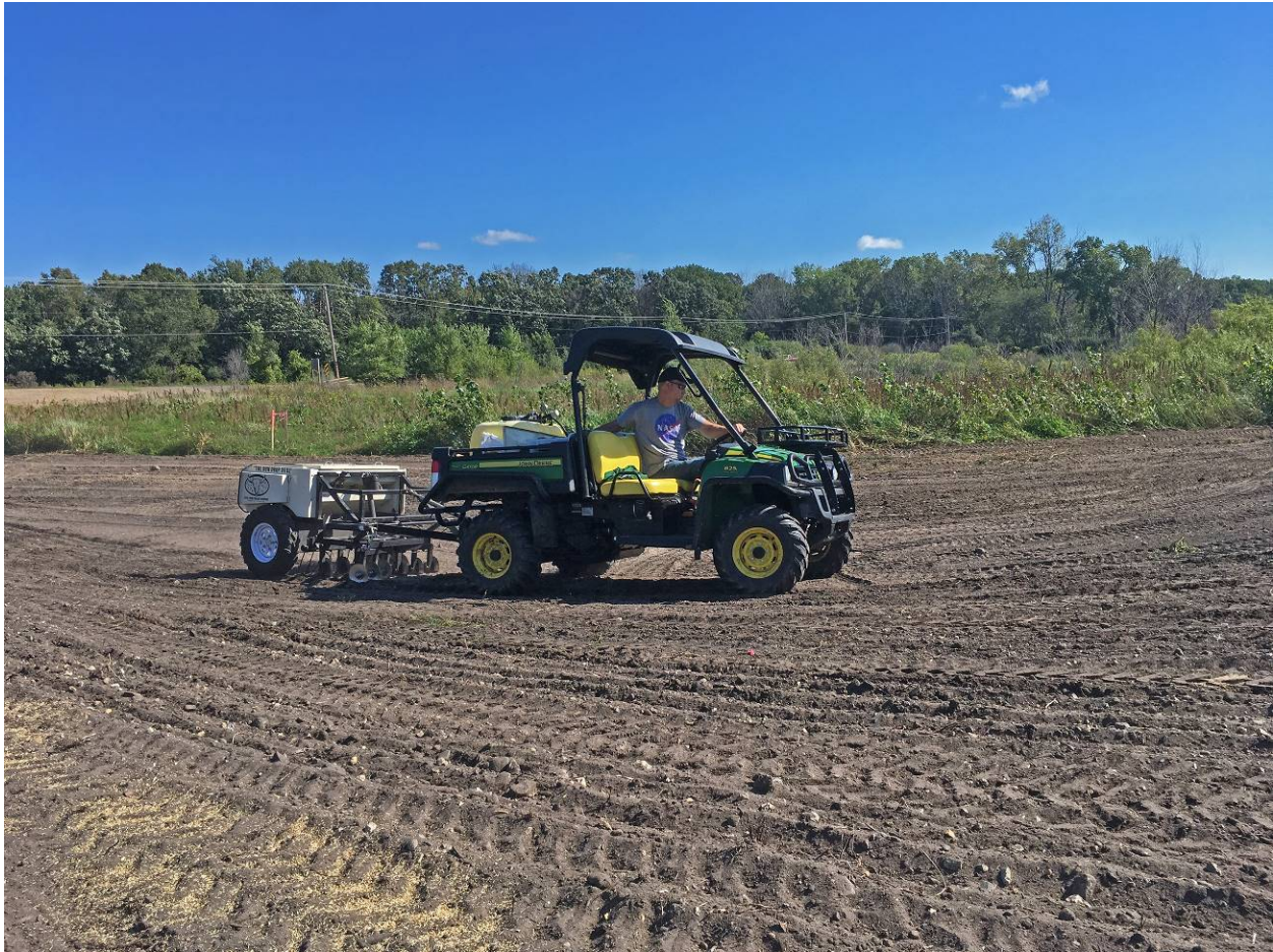
A dew drop seeder was used to install seed on the berm.
