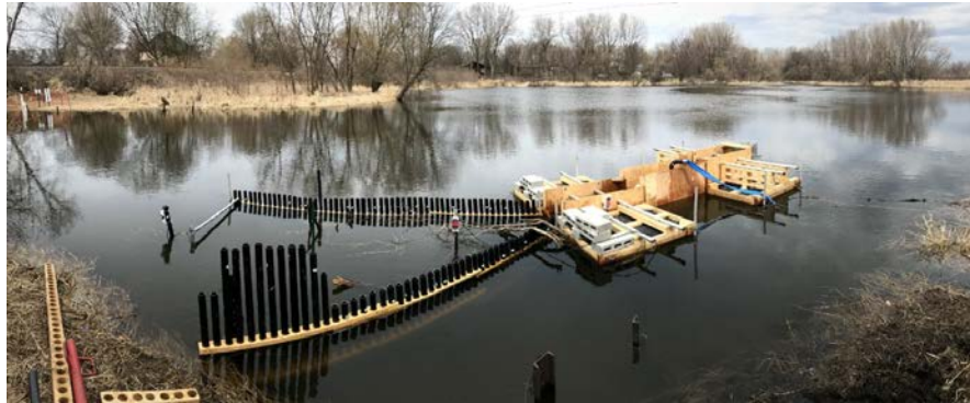
Figure 4: Carp removal system on Rice Creek (fish ladder, Whooshh System) ( https://medium.com/@MnBWSR/the-potential-application-is-huge-3789a37fa190 )
