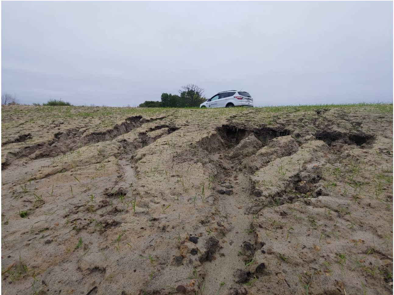
The severe rain events caused 1-2' gullies on the slopes.
