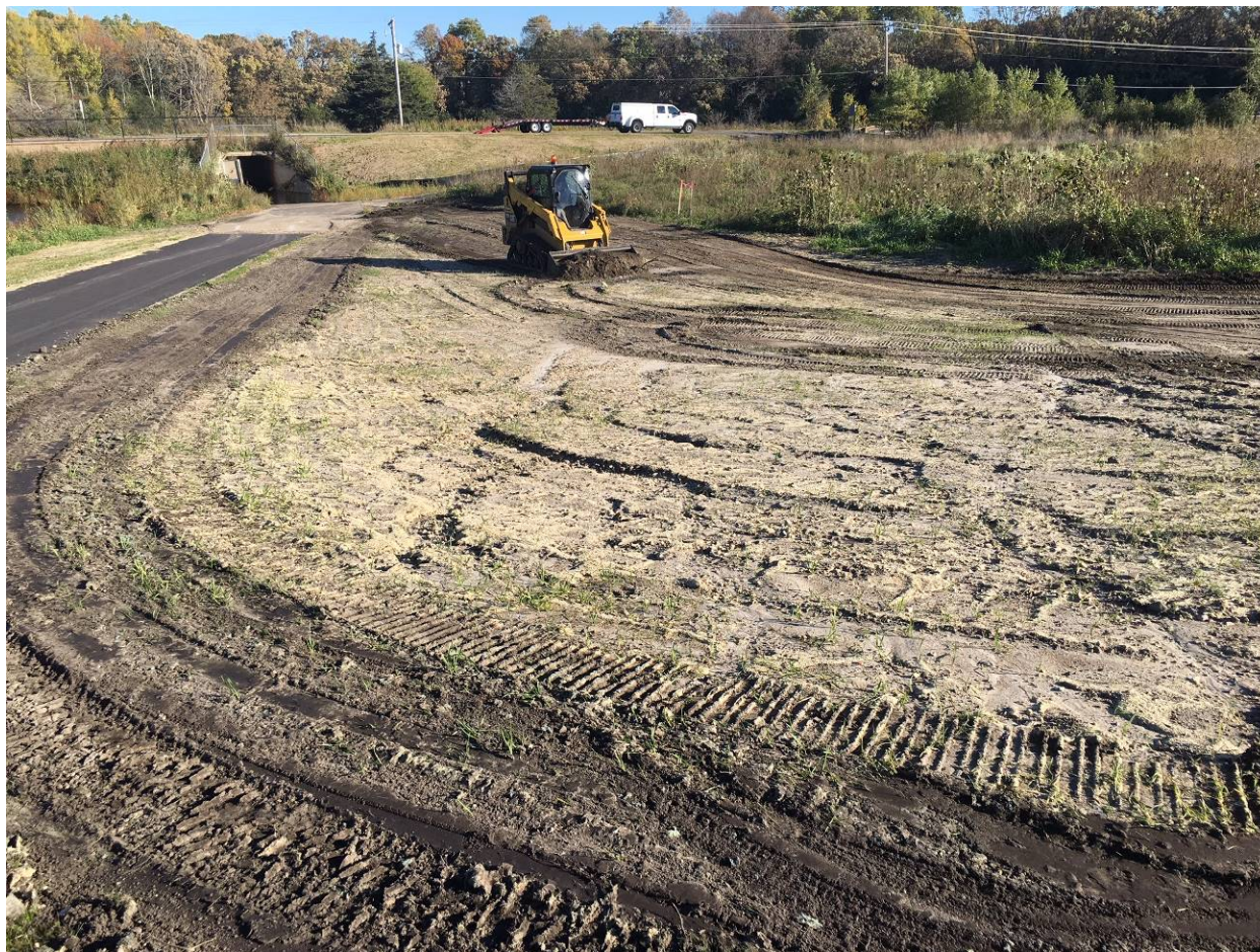
Seen from RCC re-grading the site with a skid-steer.
