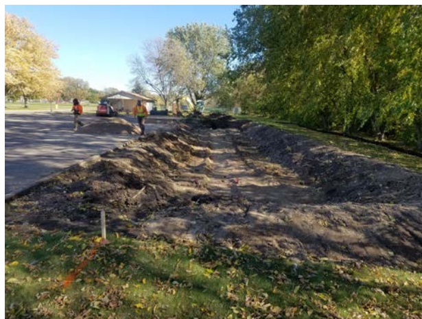
Rough grading completed at the House of Prayer rain garden in Oakdale
