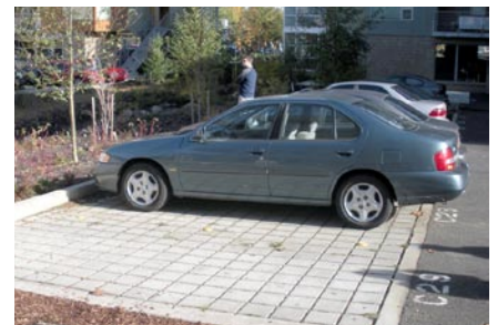
Pervious pavers installed at the Headwaters on Tryon Creek in Portland, OR.
