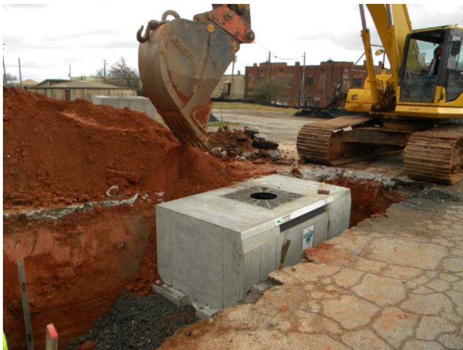
Figure 4: Installation of a BioPod™ treatment system in College Park
