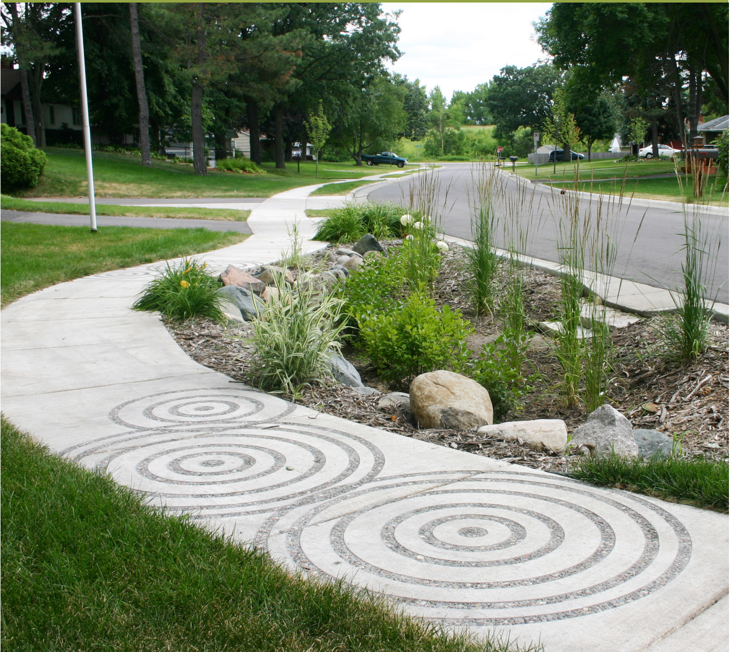
above: The City of Maplewood embraced the living streets design framework for street reconstruction projects to lower long-term costs, reduce impervious surface, and treat stormwater.
