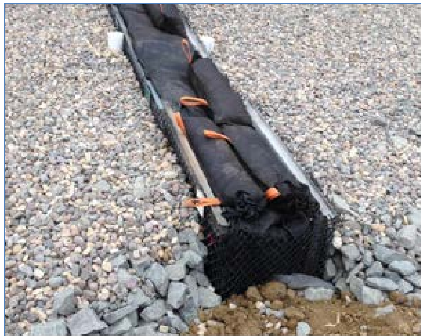
Figure 7 Photo of filter core in check dam (from Natarajan and Gulliver, 2019)
