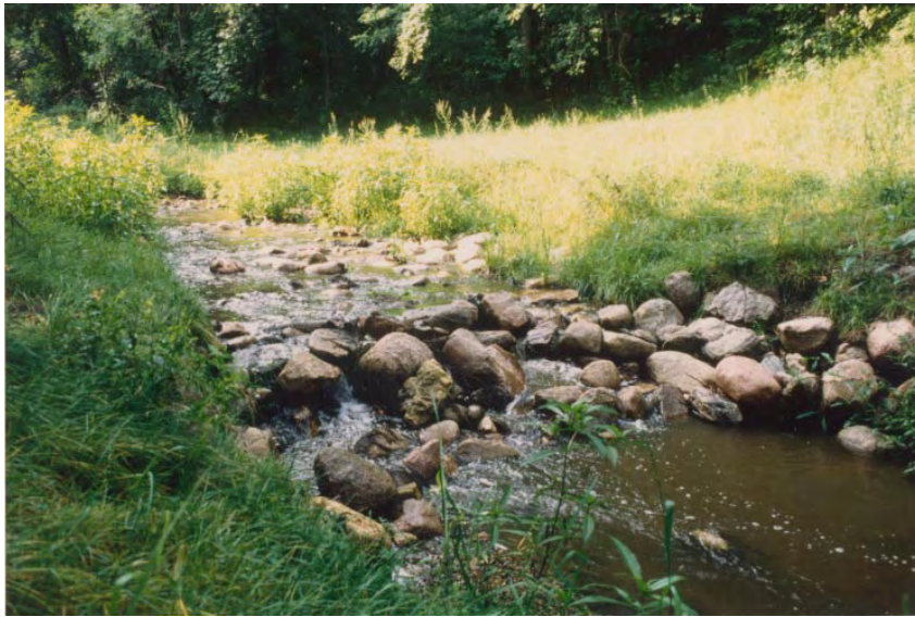
Photo 3. Rock drop structure at Battle Creek Park.
