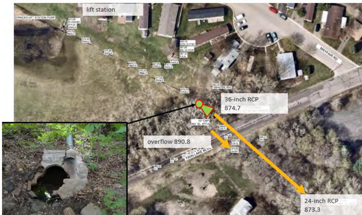
Figure 2-2 Culvert below Twin Lake Boulevard
