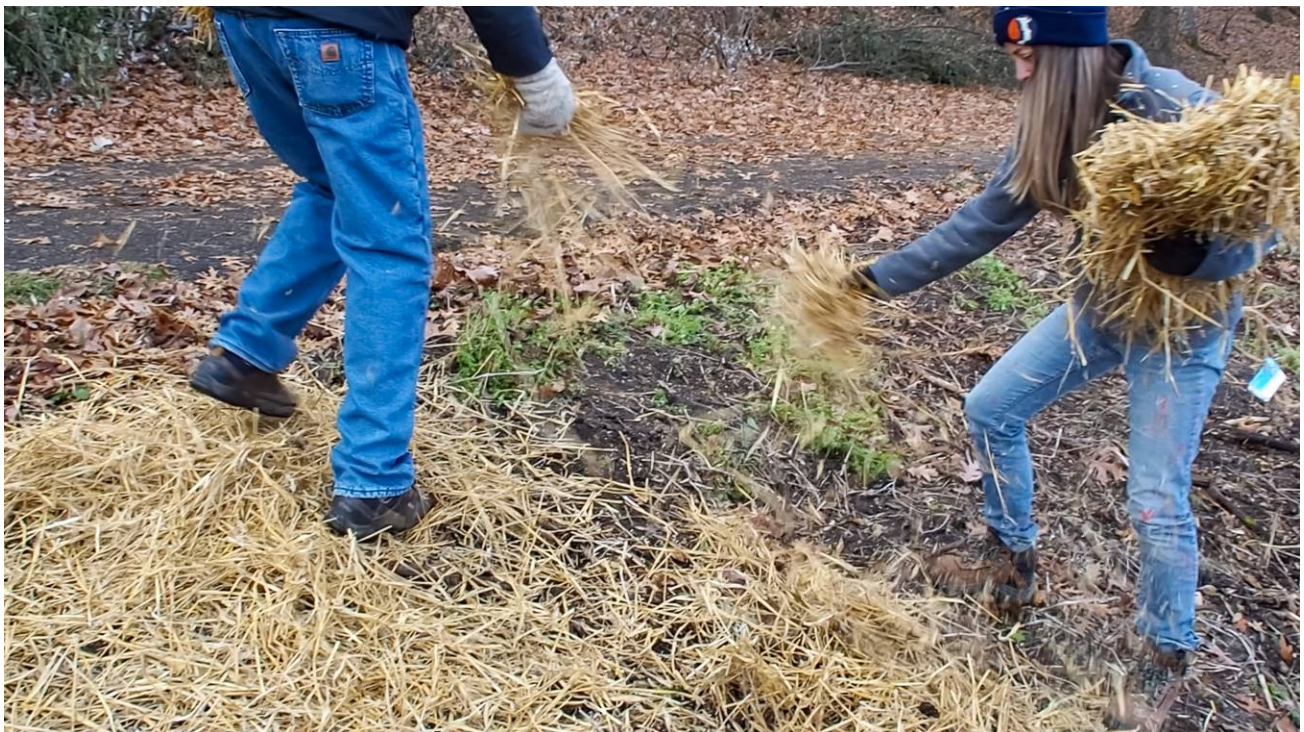
Weed free prairie straw is used to cover the newly seeded buffer areas.
