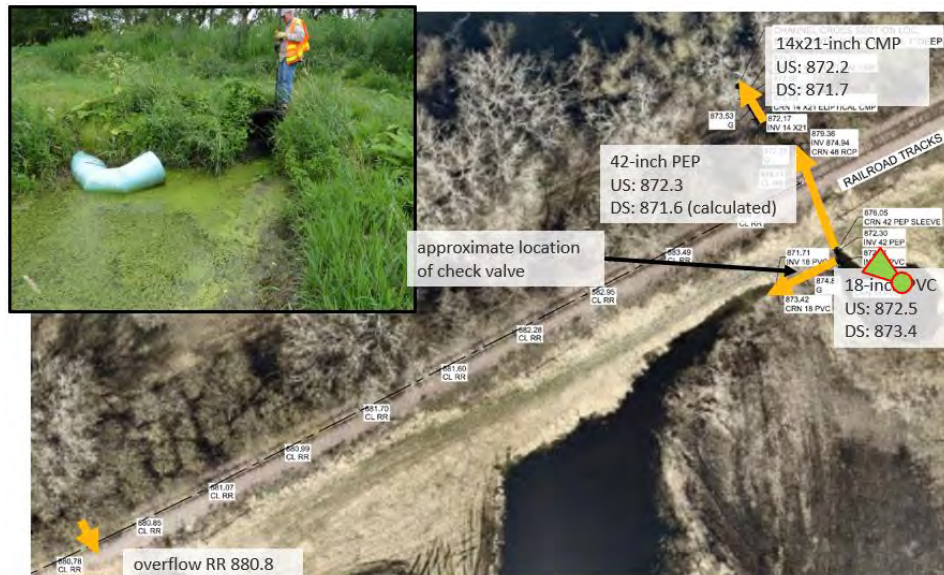
Figure 2-3 Upstream of Culvert below Railroad Tracks
