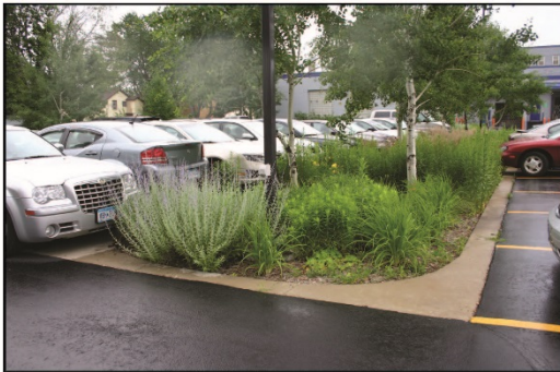
Commercial Parking Lot Rainwater Garden 7-Sigma Manufacturing, Minneapolis
