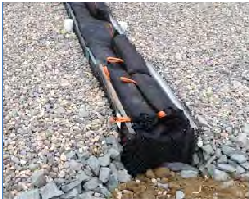
Figure 7 Photo of filter core in check dam (from Natarajan and Gulliver, 2019)
