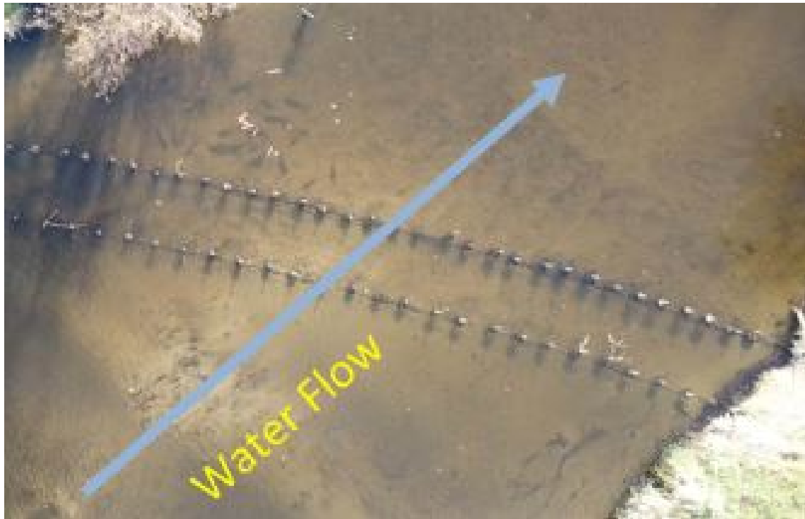
Two strips of low voltage electrodes on the bottom substrate compose the barrier on Rice Creek.
