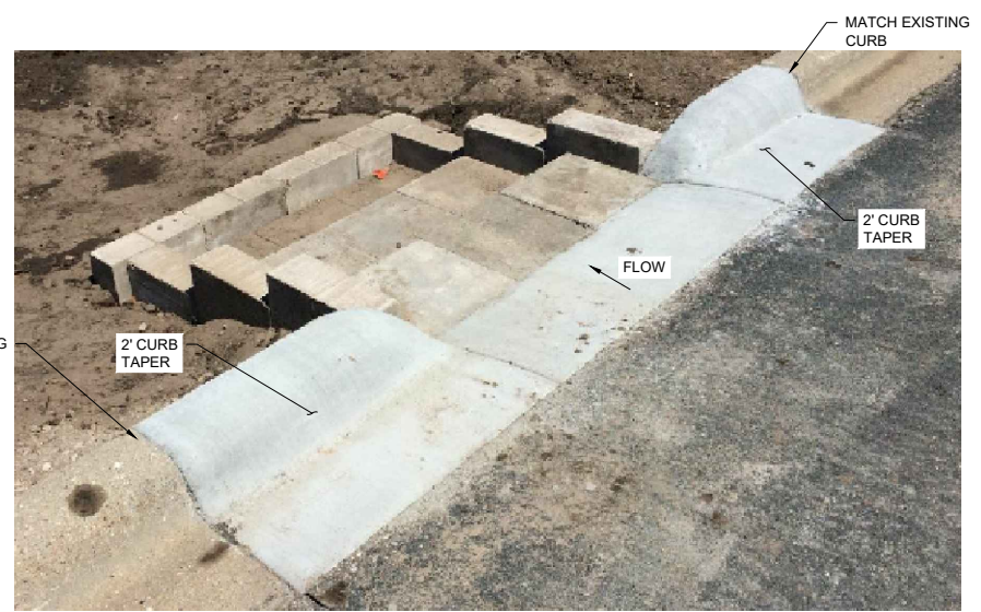
4 DETAIL: SPLASHBLOCK ASSEMBLY EXAMPLE
