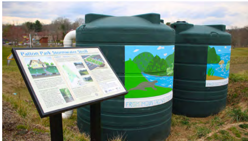
Figure 2: Rainwater cisterns with an educational sign from the Patton Park Stormwater Stroll
