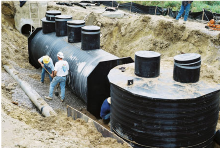
Figure 5: installation of the AquaSwirl and AquaFilter components
