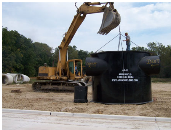
Figure 3: AquaSwirl installation
