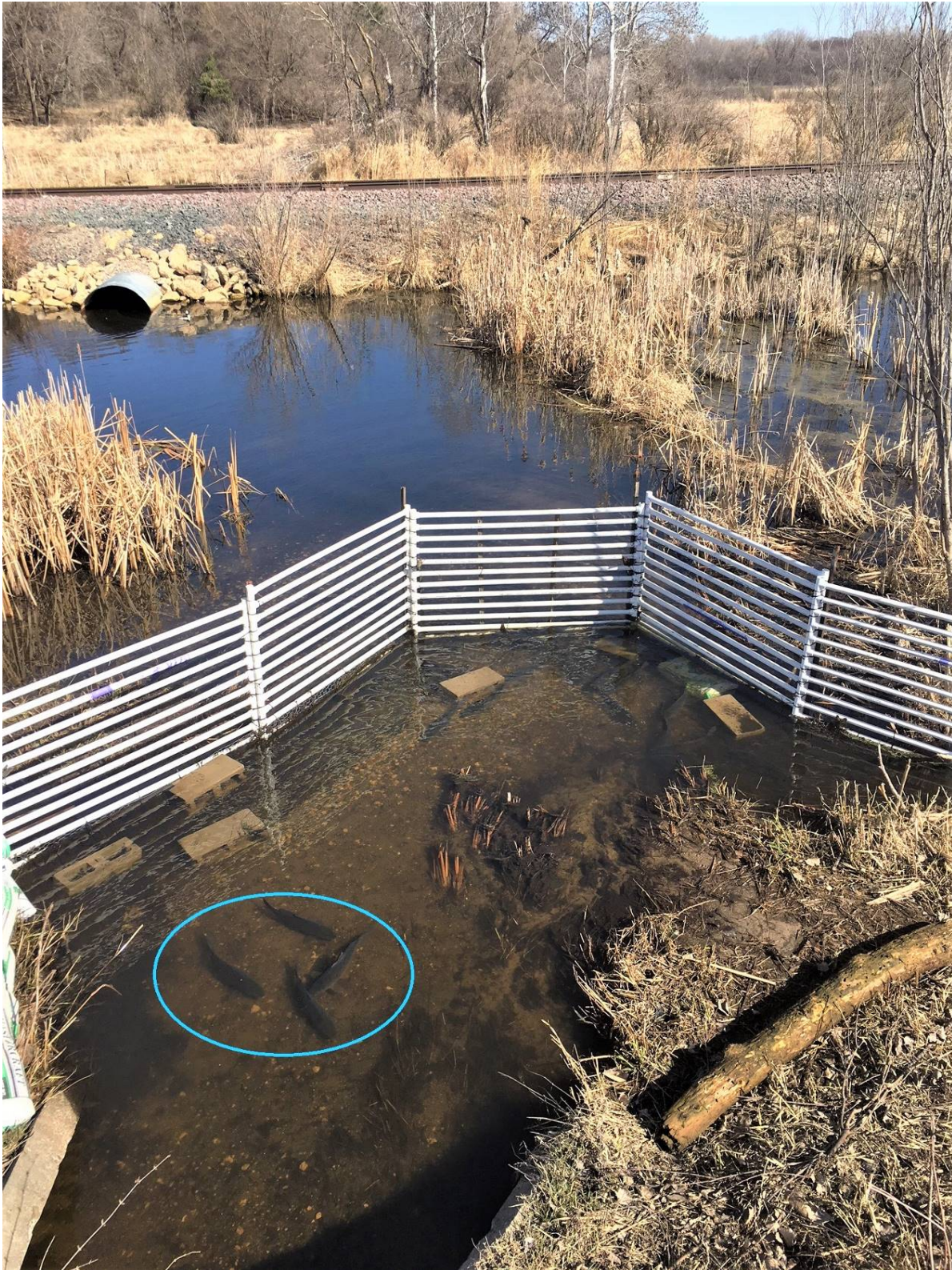
This barrier is preventing carp from moving into a wetland complex just south of Lake Owasso. The blue circle is highlighting four common carp.
