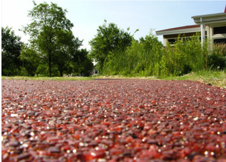
Figure 5: Prairie Crossing School FilterPave sidewalk
