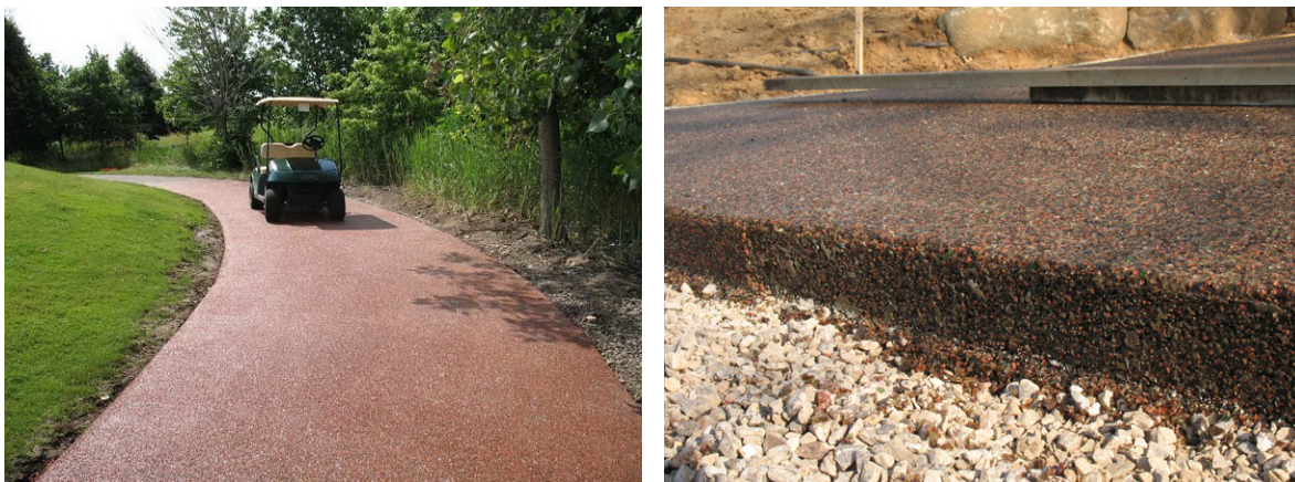
Figure 1: FilterPave slab and golf cart path application
