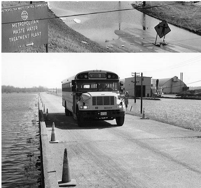
Top: School bus transports workers from the plant to remote parking areas via a temporary gravel road crossing flooded Childs Road during spring 1997. Bottom: At peak, the 1997 floodwaters approached the concrete surface that tops the sanitary sewers carrying wastewater into the plant.
